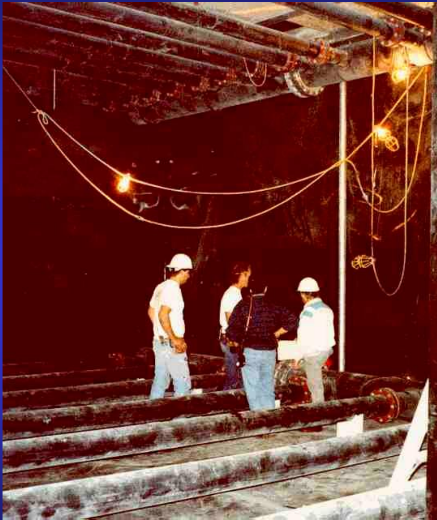
10,000 ton hours - concrete tank
