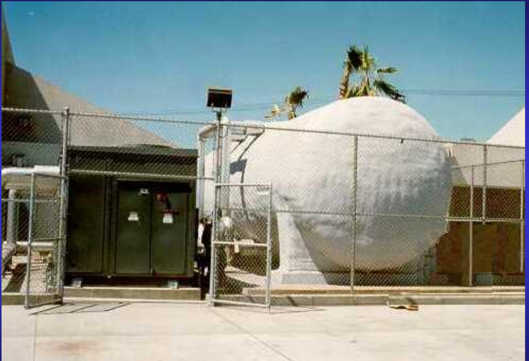
Completed Tank with Urethane Foam Insulation
