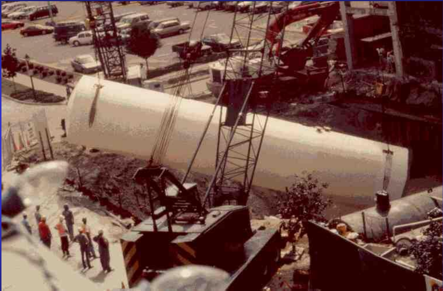
Horizontal Pressure Vessels for Direct Burial
