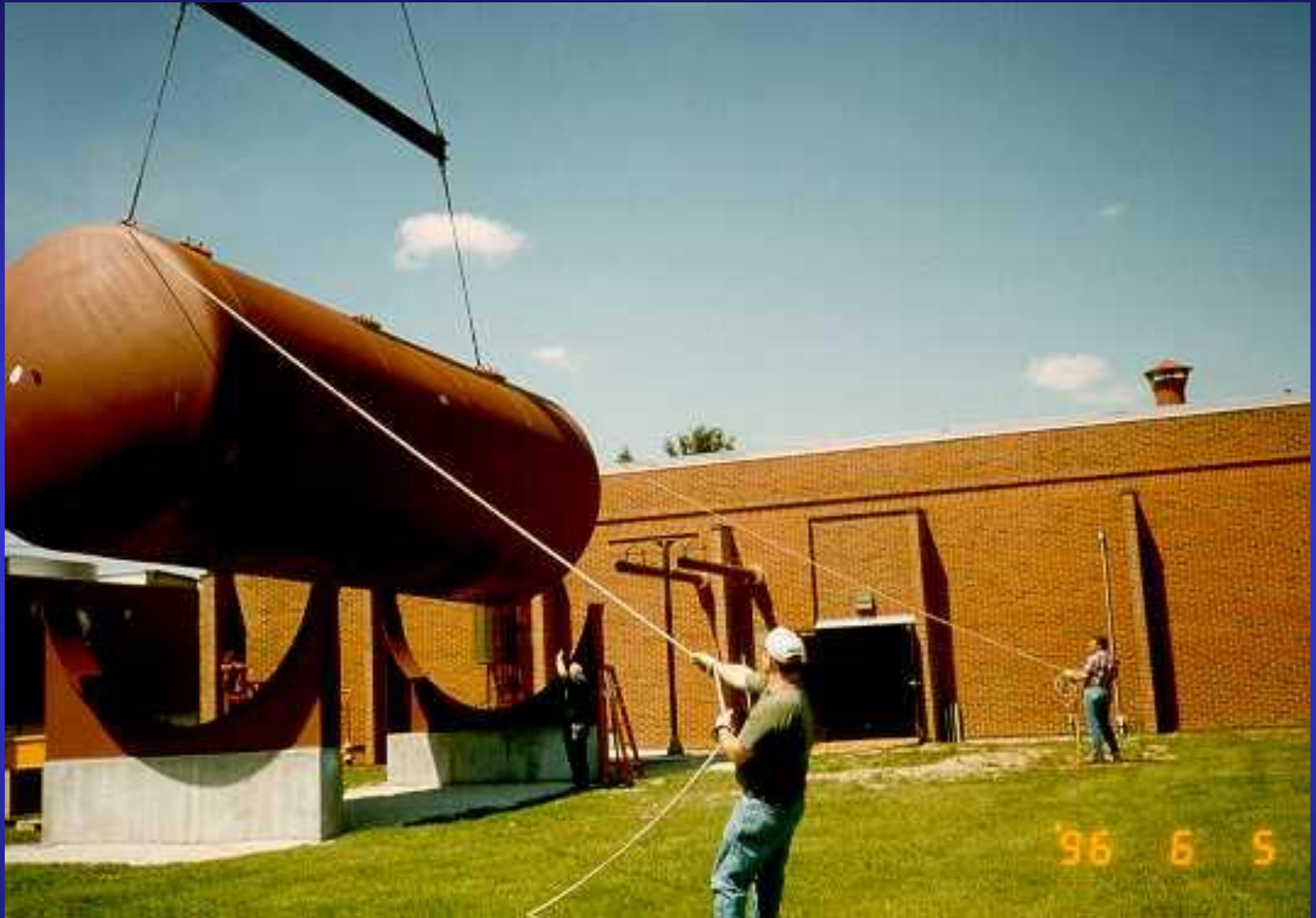
Setting Tank in Saddles - Minimum Foundation Concrete Required
