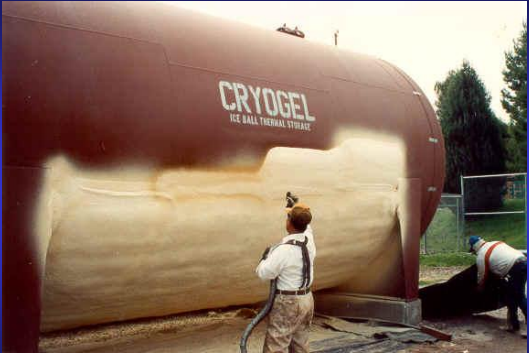
Urethane Foam Insulation Sprayed Directly onto Tank
