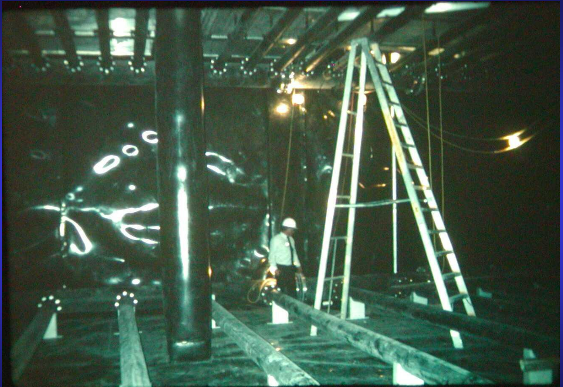
Polyethylene Liner in Concrete Tank
