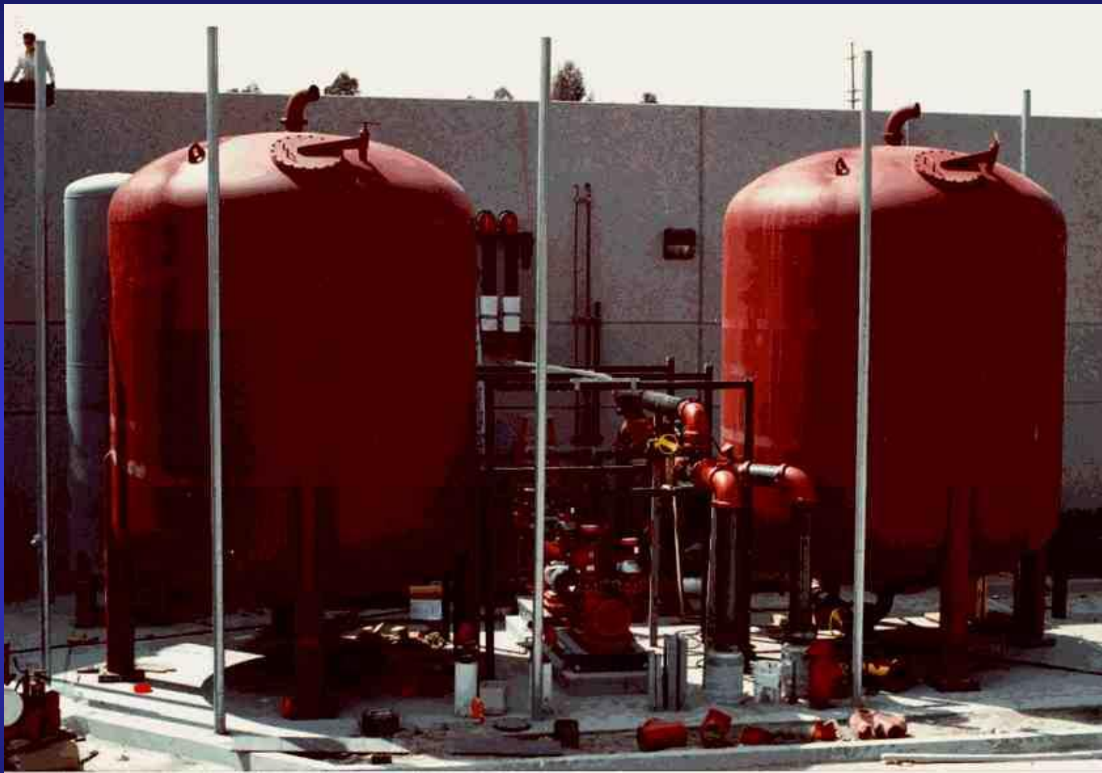
Vertical Pressure Vessels - Minimum Space and Height
