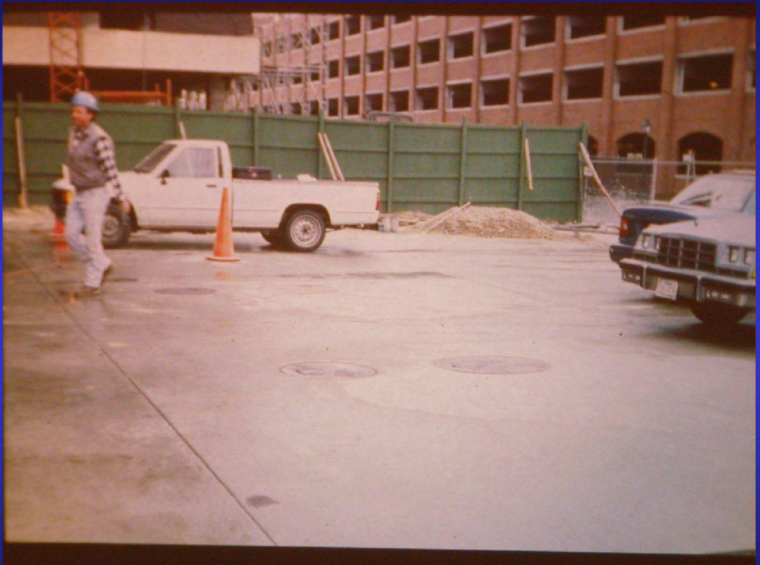
Finished Project - Underground Tanks - Only Manways are Visible
