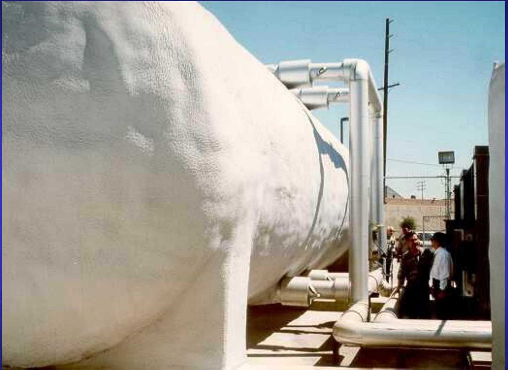
Tanks Fully Insulated with Urethane Foam and UV Top Coat
