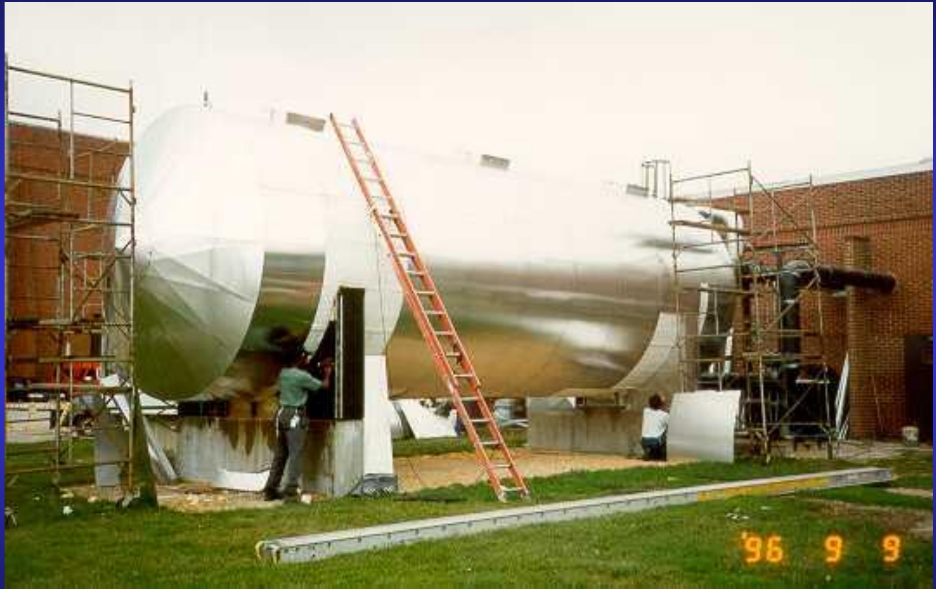
Final Insulation and Jacket Installed
