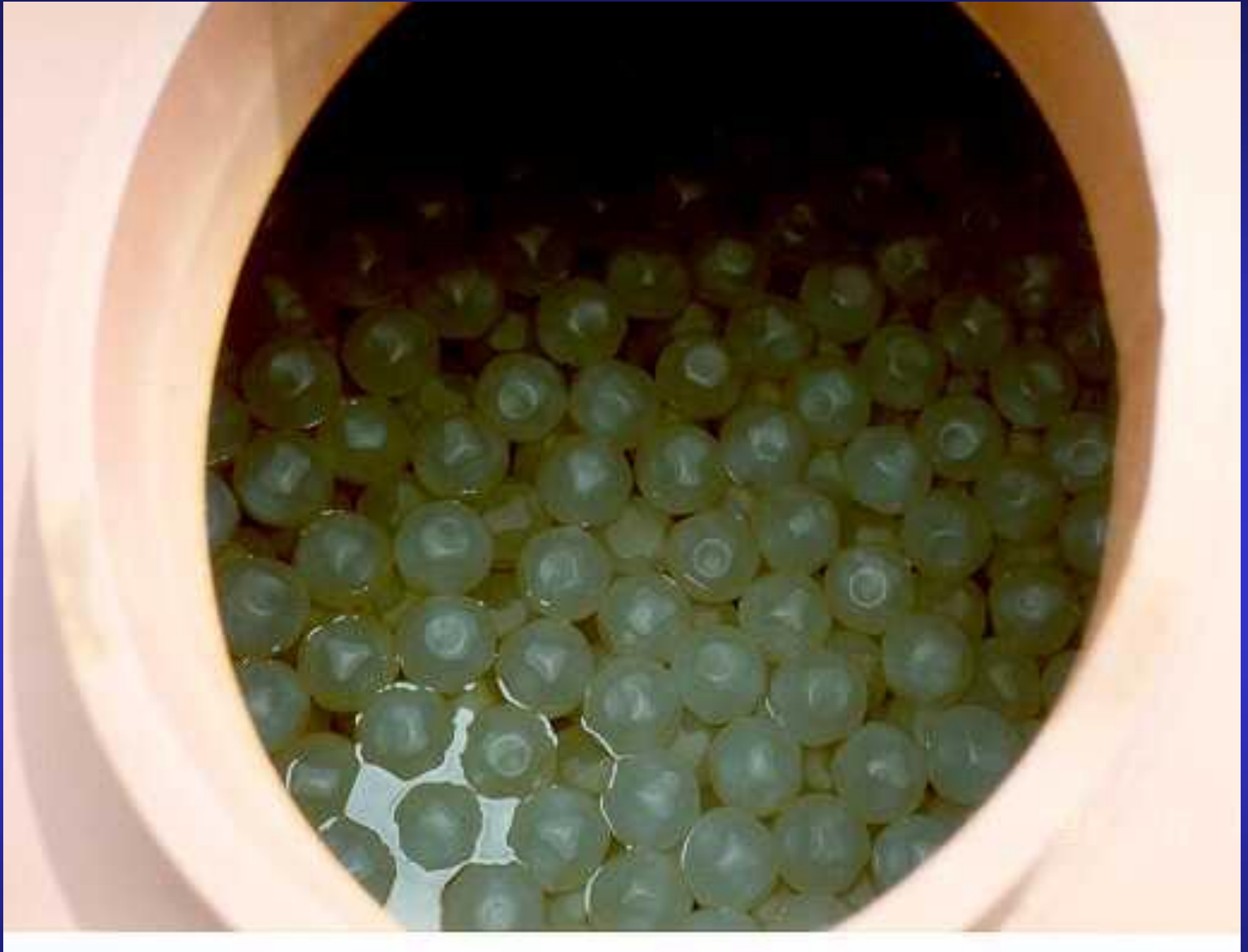
Ice Balls Floating in Water - - Water Assist by Breaking the fall of the Balls Balls Float to Spread Out Through the Length of the Tank
