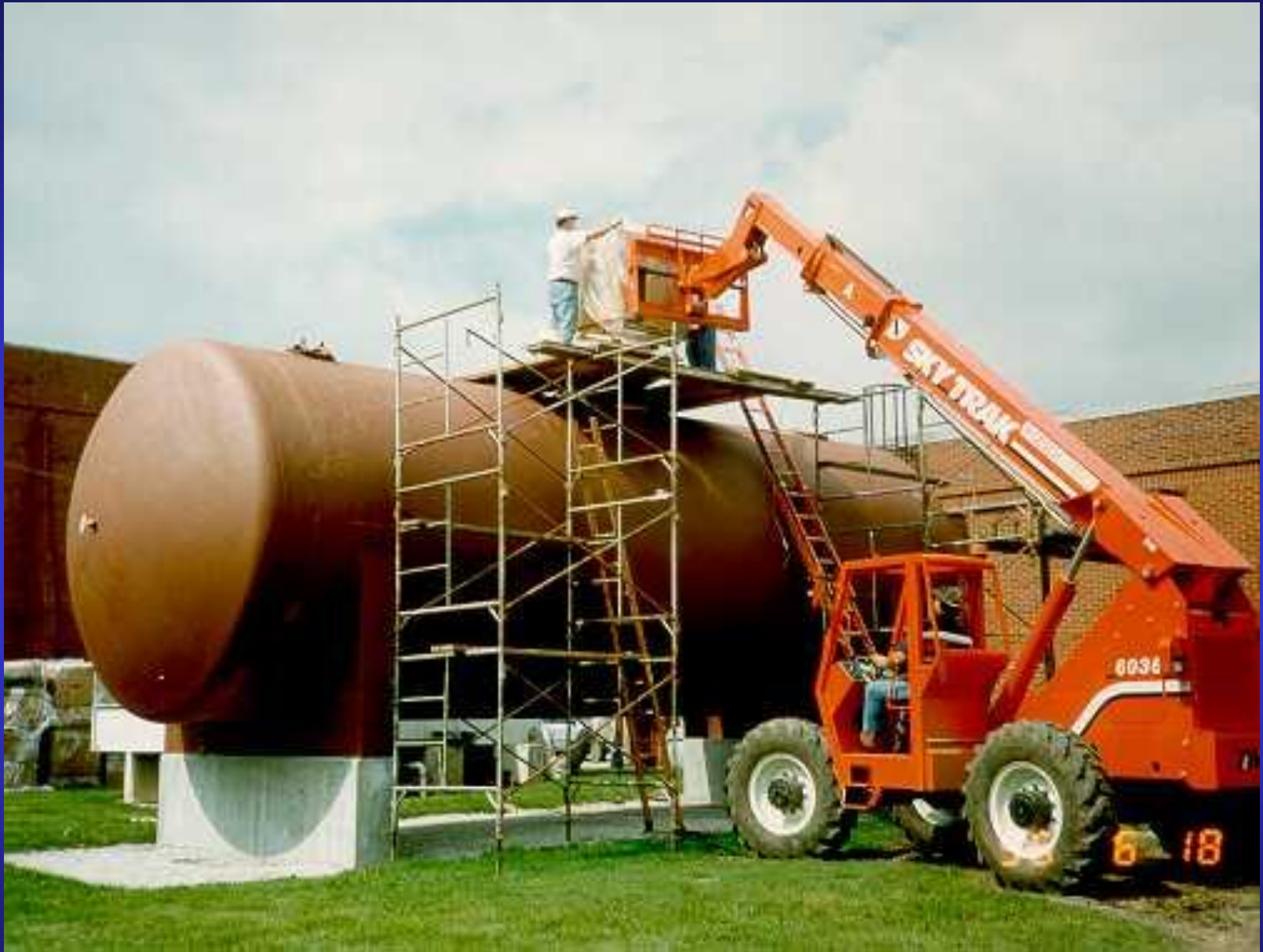
Raising Ice Balls Freight Container to Top of Tank
